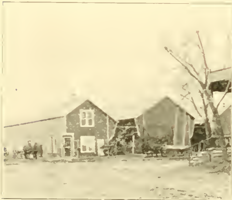
CHICAGO LUMBER COMPANY'S YARDS AT GLASCO.
